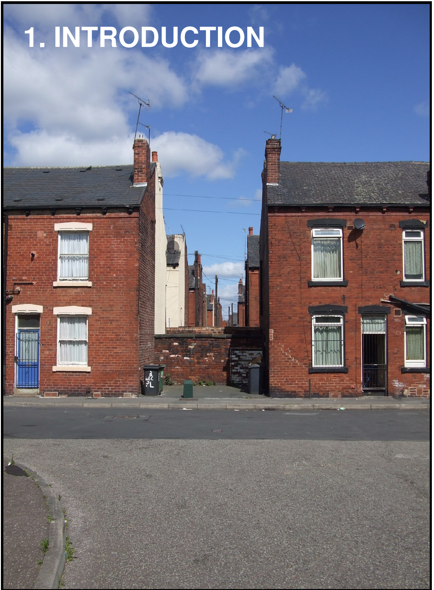
View through the bin yards from Recreation Street to Brown Lane East, Holbeck, Leeds.
