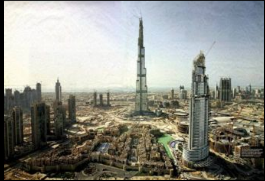
Al Burj, Dubai – every m 2 floor space needs 1.5m 3 concrete to hold it up (Simon Smith) The Shard – Ancient or Modern?
