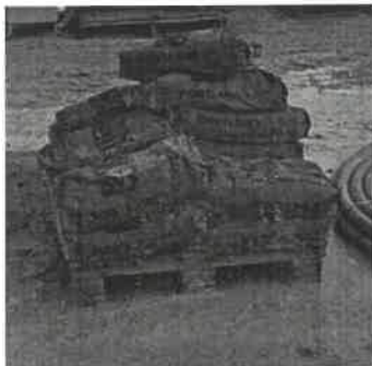
Water-logged pallet of cement bags
